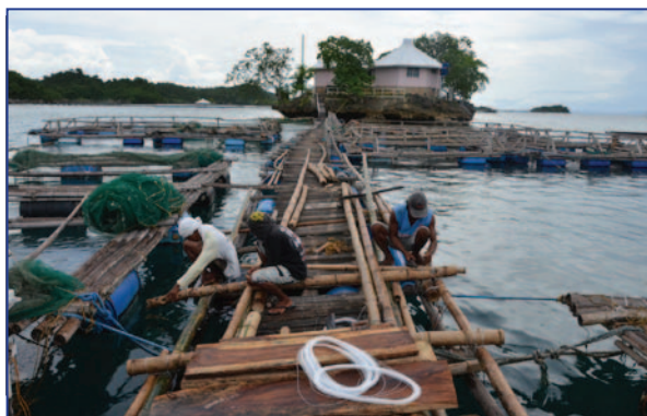
Figure 7: Mending and maintenance of bamboo frames
