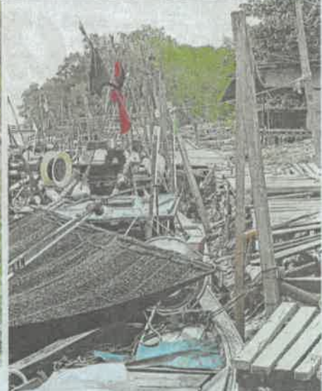
The jetties at Pengkalan Kanchong Laut are unsafe and need improvement.
